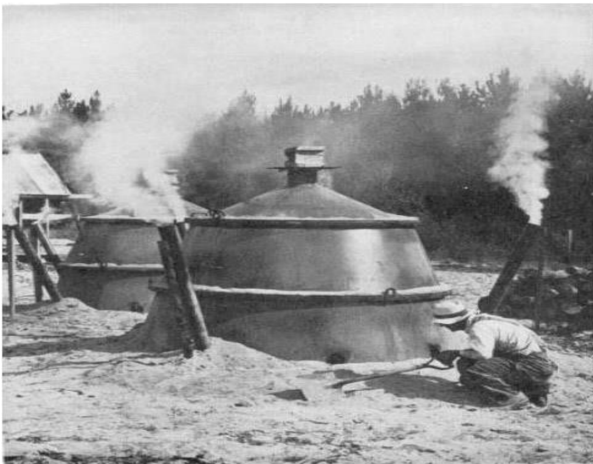
Portable, sectional sheet-metal kiln.
