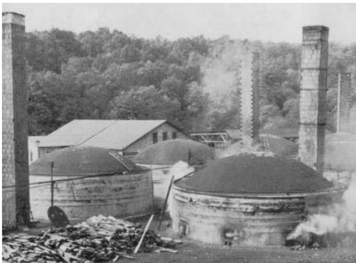
-Ceramic kilns converted for charcoal manufacture.
