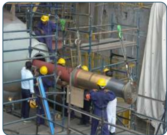
Shaft line installation
