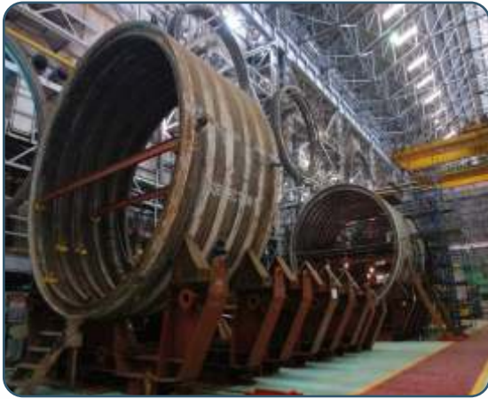
Fabrication of sections
