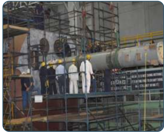
Installation of torpedo tubes
