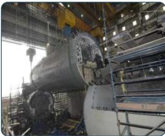
Lowering of sections on pontoon
