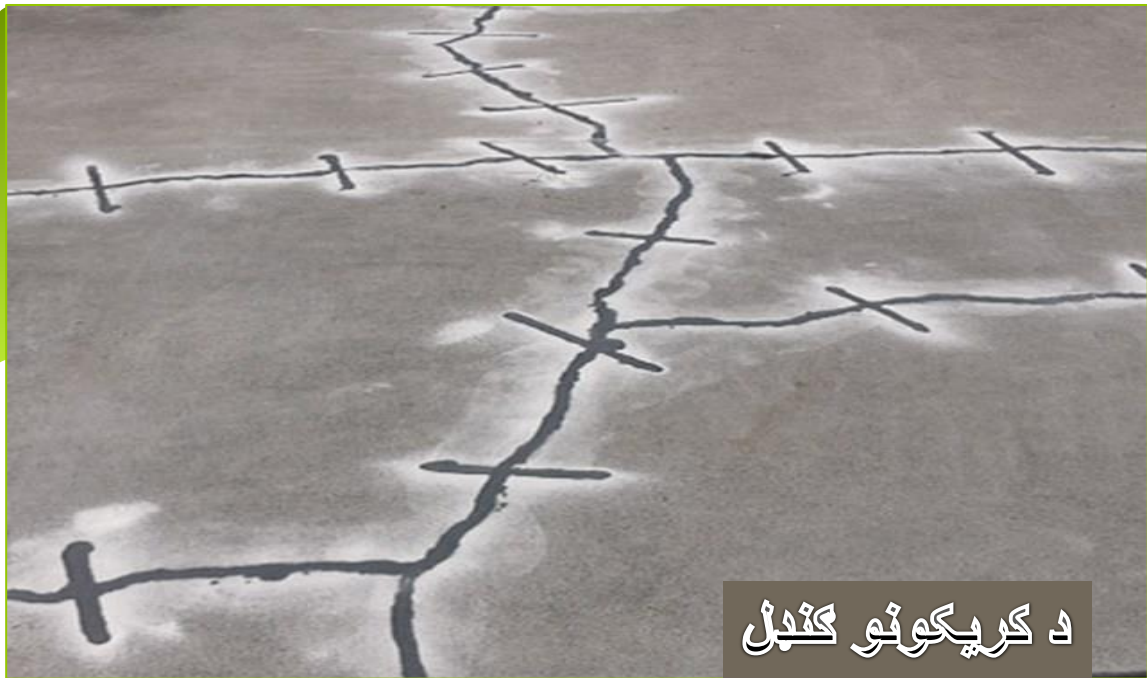
Figure 3: Stitching & Doweling
