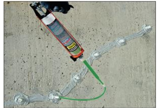
Figure 3. High pressure Injection Pump
