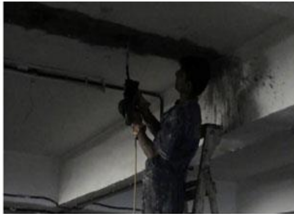
Figure 5. Epoxy injection in progress
