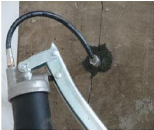
Figure 4. Injecting with a hand pump
