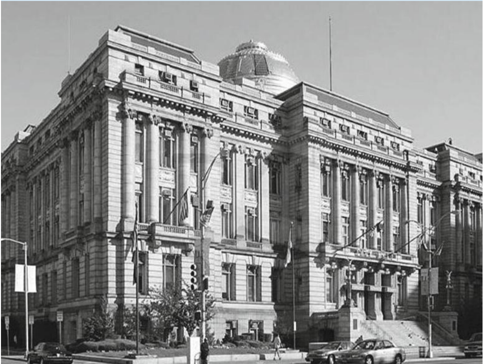
Newark City Hall, Newark, New Jersey
